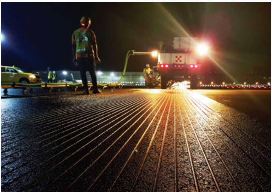
Trapezoidal grooving was added to the newly resurfaced Runway 1 to enhance aircraft tyre grip and lower the risk of skidding by planes.
